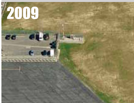
Block Island, RI , adjacent to parking lot and aircraft parking area. RATING = CRN4
