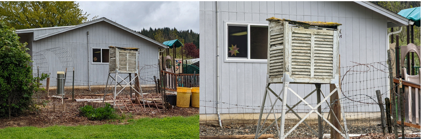
CRS placement at rear of Cooperative Observer's residence at Elkton, ID. Note the deterioration of the CRS, including rot, mold, and peeling paint. Observations are still taken daily here. Source: Anthony Watts.
