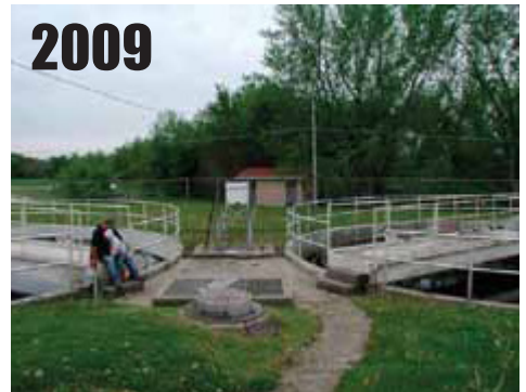
Morrison, IL , sited on concrete, between open wastewater tanks at WWTP. RATING = CRN5
