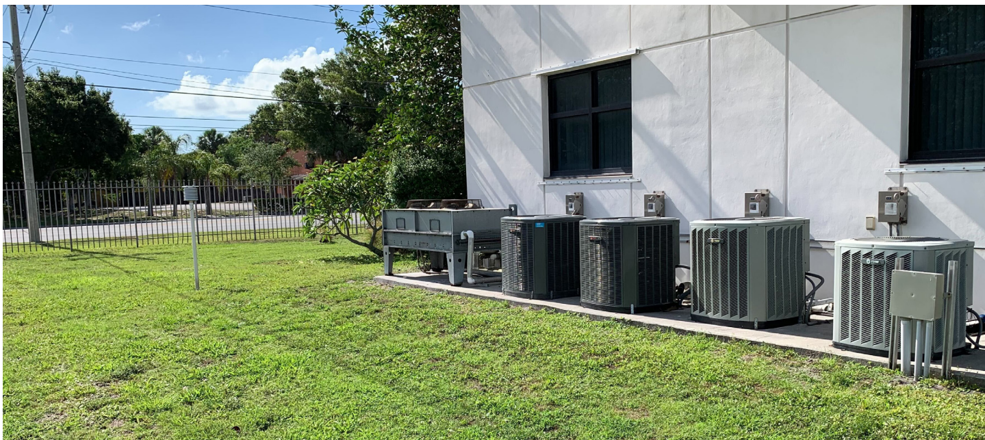
MMTS placement near a building and five air conditioner units at a WWTP, a GHCN station in Fort Pierce, FL. The a/c units produce waste heat, which can easily bias the sensor warmer. Source: Tim Benson.
