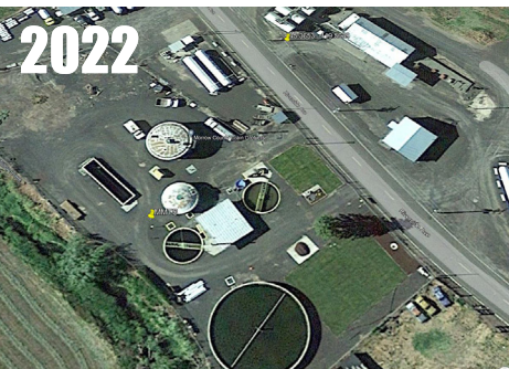
No change in location. Unable to ground survey. RATING = CRN5
