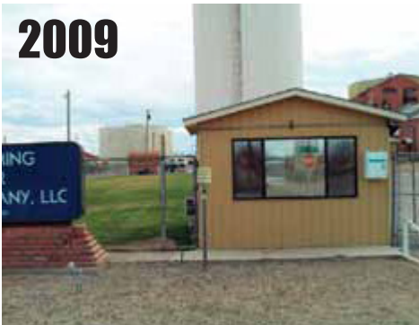
Worland, WY , nearby sidewalk, brick sign mount, gravel at base, outbuilding. RATING = CRN4
