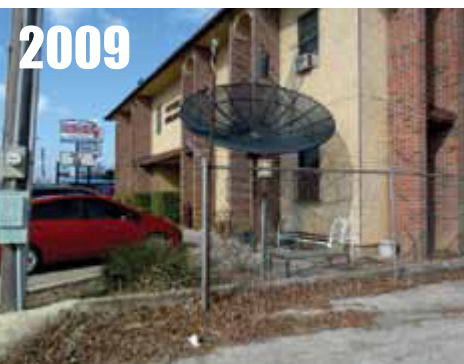
Lampasas, TX , next to sidewalk, near satellite dish, road, parking lot, building. RATING = CRN5
