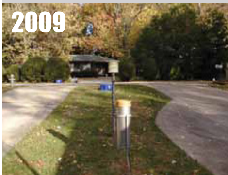
Gainesville, GA , between two driveways. RATING = CRN4
