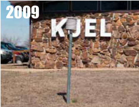
Lebanon, MO, nearby radio station building. RATING = CRN4
