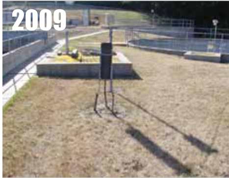
Winnepago, MN , at city WWTP, nearby sewage tanks, concrete pad. RATING = CRN4
