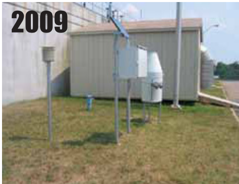
Staunton, VA , at WWTP, between tank wall and paved road. RATING = CRN4
