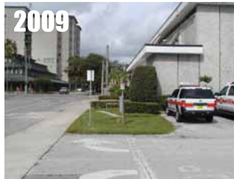
Bartow, FL , nearby building, road, parking lot. RATING = CRN5
