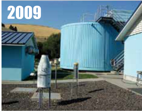
Dayton, WA. Water plant, over cinder rock, near vents, buildings.
