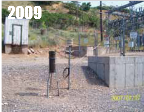
Spanish Fork, UT , sited on gravel, near concrete wall at power station. RATING = CRN4
