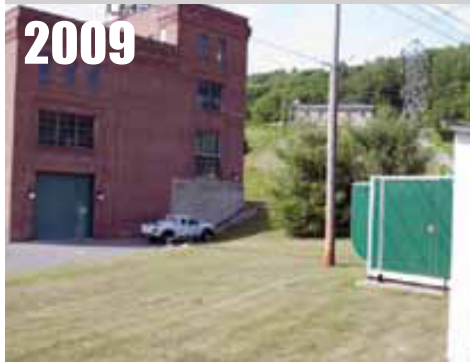
Falls Village, CT , nearby building and parking lot. RATING = CRN4
