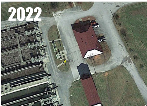
No change. Unable to get access for ground survey. RATING = CRN5
