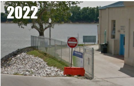
Location unchanged, but ironwork has been removed and replaced by chain-link fence. RATING = CRN4
