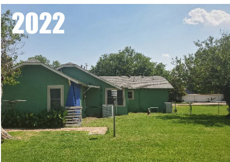
Location moved, but now near sidewalk and A/C unit, building. RATING = CRN4
