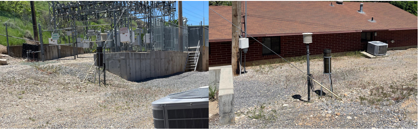
MMTC placement at USHCN station in Spanish Fork, UT. Note the a/c unit and the power substation. Also note the proximity of the roof, due to the thermometer's elevation. The location is at a power generation facility. Source: Steve Randle and Ron Broadway.
