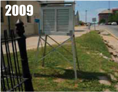
Mount Vernon, IN , nearby road, building, ironwork. RATING = CRN4
